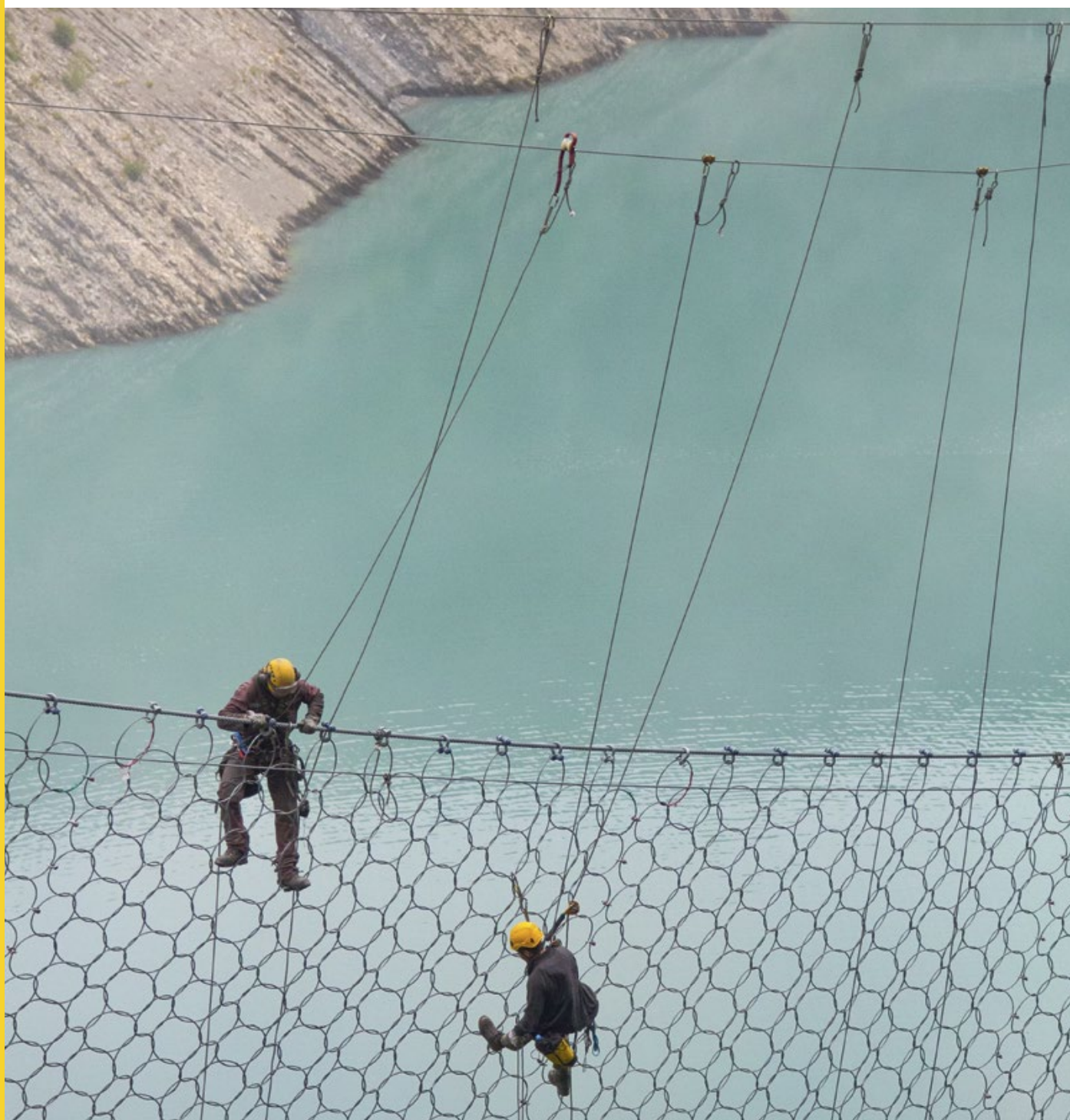
Road protection works, Chambon dam, France. © vuedici.org / Hydrokarst / Département de l'Isère
