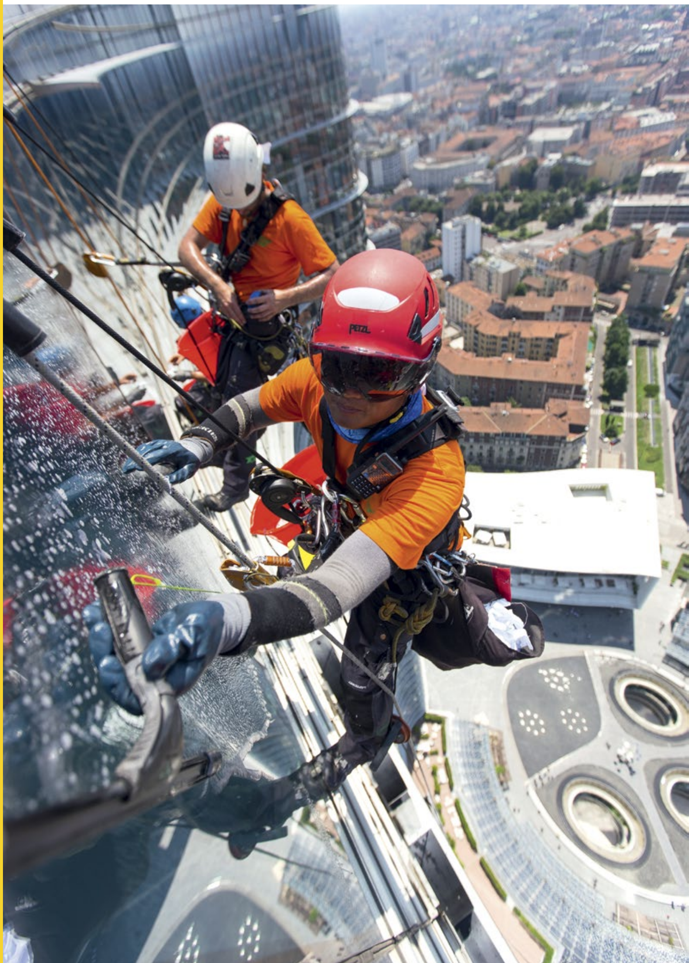
Window washing Unicredit Tower A, Milano, Italy. © Petzl / vuedici.org / Unicredit Tower A / Rigger Italia
